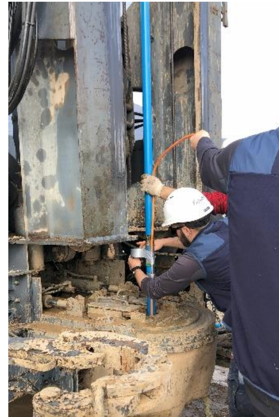
Electrodes array installed in PITOP5
